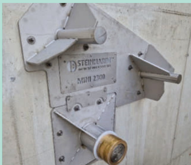
Rotating bearing for the HydroSlide® outflow control system, Flood Control Reservoir Rettenbach, Sölden, Tirol
