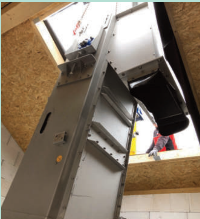
Assembly of the FSM Multi Rake Bar Screen and the FSM Screening washing press
