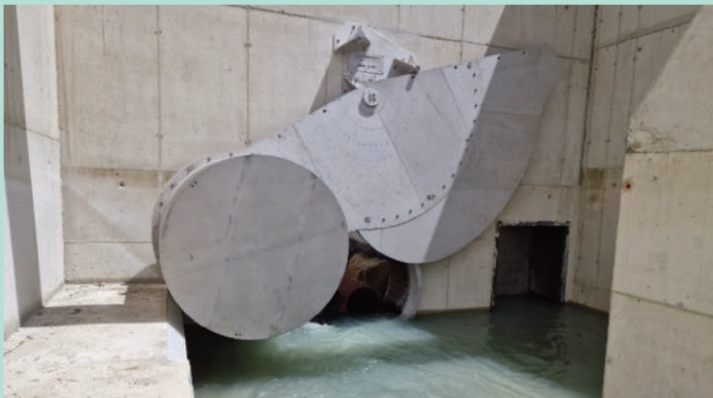
Test (maximum reduction) (l.) and operation (not dammed) (r.) of the Steinhardt HydroSlide® outflow control system DR 2300 – Flood Control Reservoir Rettenbach, Sölden, Tirol
